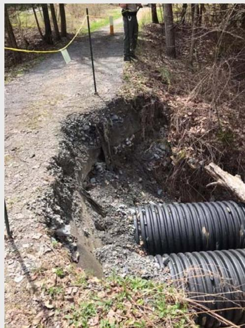
After the flood, culvert pipes were exposed where a section of the Overlook Trail was washed away.
