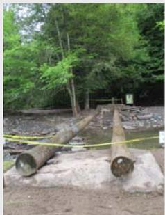
Major progress has been made on the **footbridge**. The state's "swing crew" — the work crew that does the jobs in the region's state parks that require large equipment — has been here for a couple weeks installing our new septic system. Before they left they put the poles in place that the decking and rails will be attached to.
