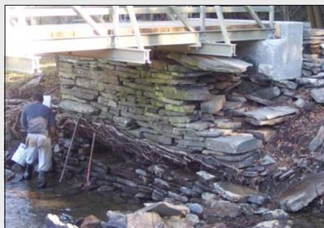
Stone abutment under the foot bridge being repaired, November 9.
